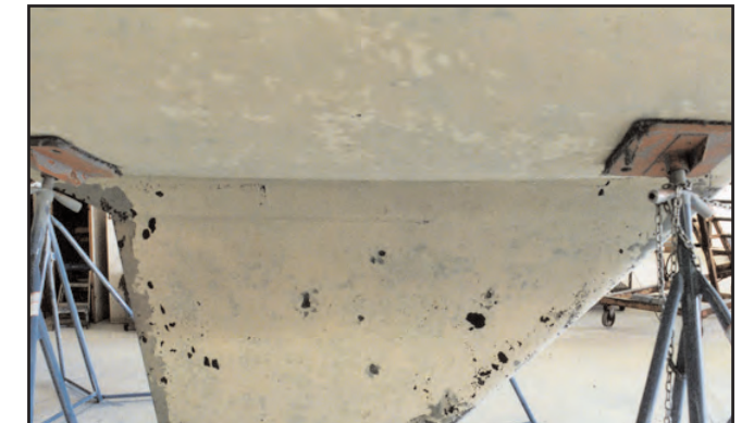
Hull ready for painting
